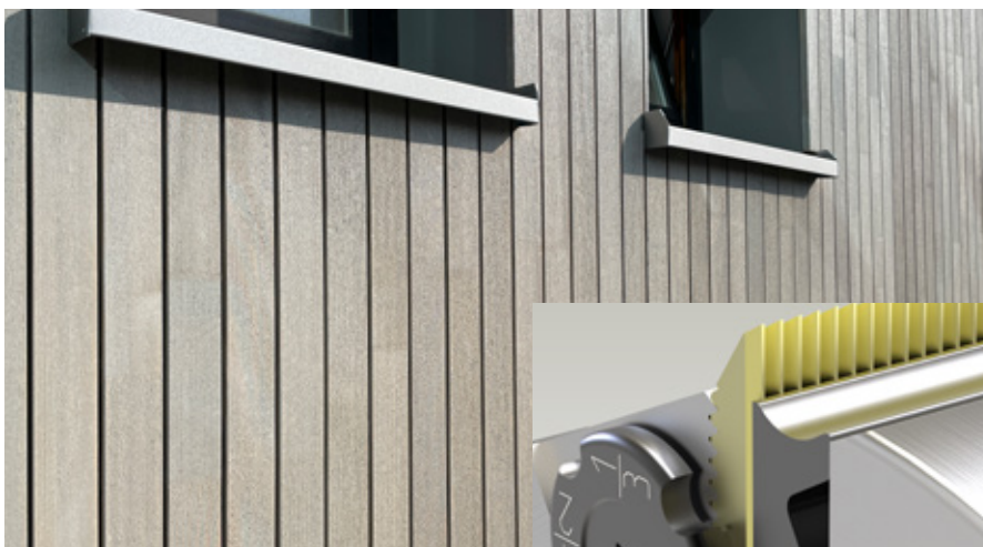
The use of profile planing knives produces facade cladding with a rough-sawn look.
